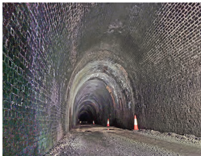
Nelson tunnel. Photo Adrian Armishaw
